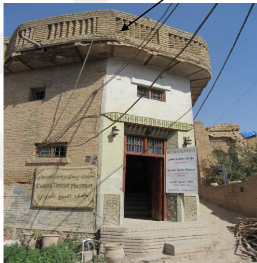
Figure 96 House Parapet in Erbil
