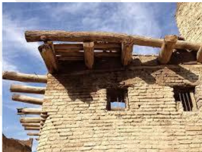
Figure 98 Brick- Basic Building Material in Traditional Period - Erbil City [70]
