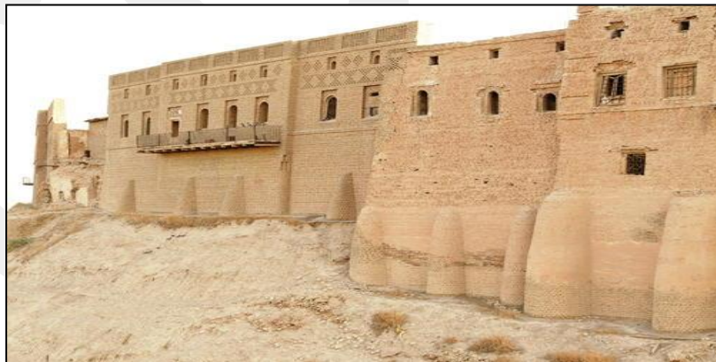
Figure 77 External Erbil Citadel Wall with Windows and Balcony [86]
