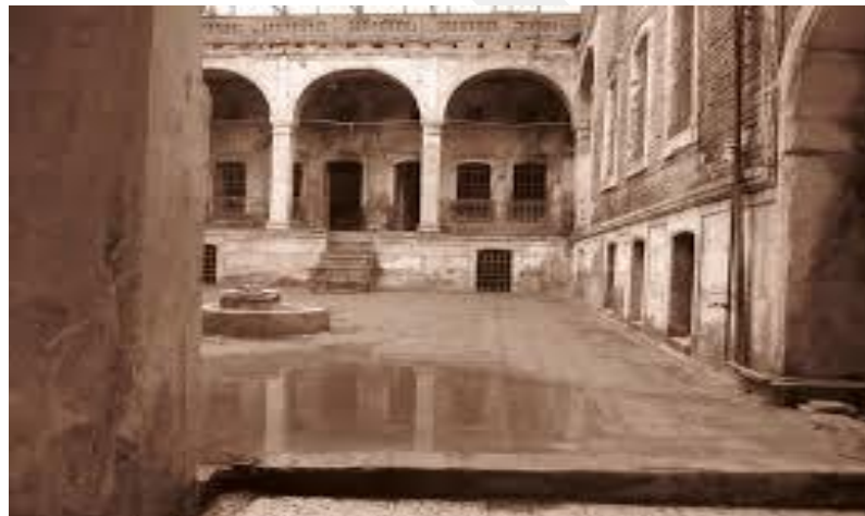
Figure 50 The Central Courtyard which has Lower Windows and Upper Windows to Let More Day Light [111]
