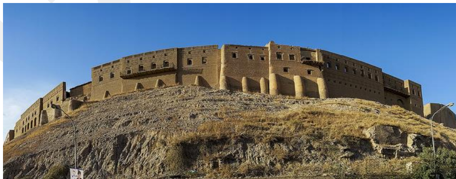
Figure 47 Erbil Citadel, All Windows or Openings on the Upper External Walls [80].
