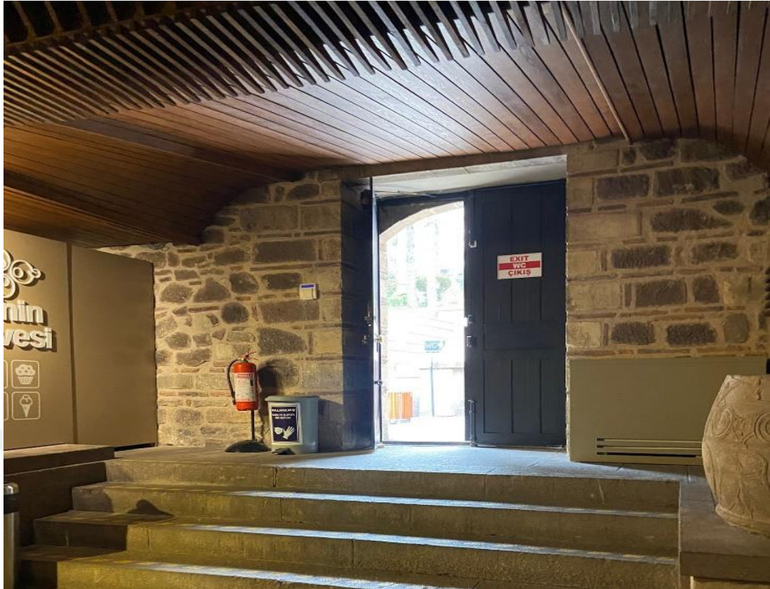
Figure 43: The exit door located next to the store.
