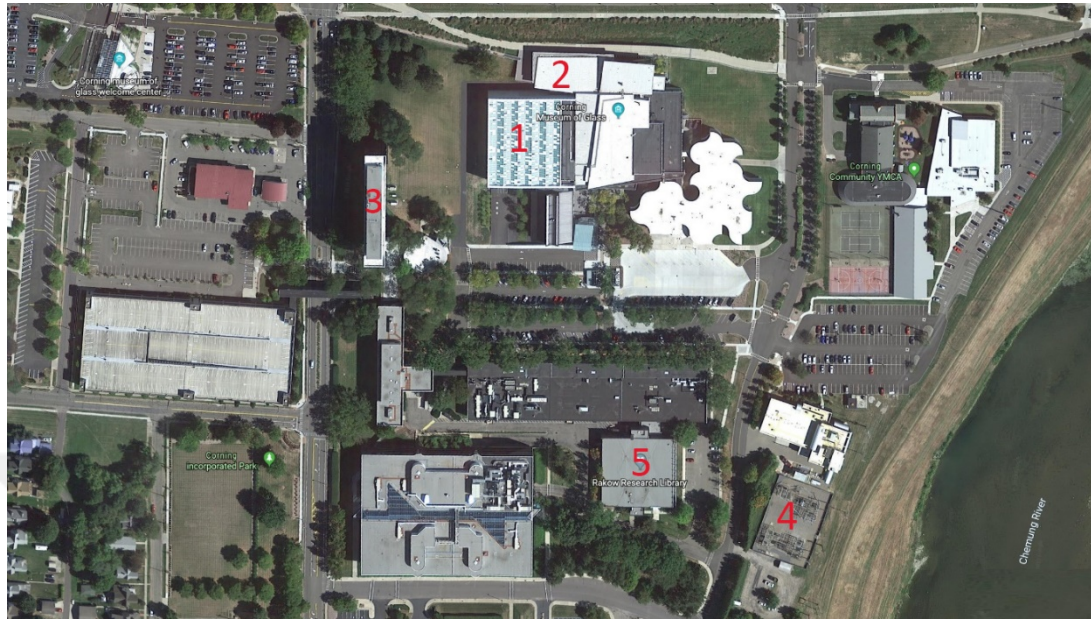
Figure 4.1: Aerial View of the CMOG
