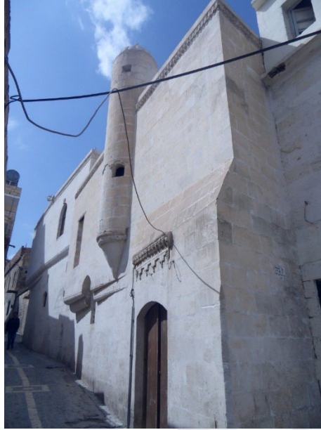
Figure 16: Nuran Elçi mansion south facade (TEMA 2008: 20)
