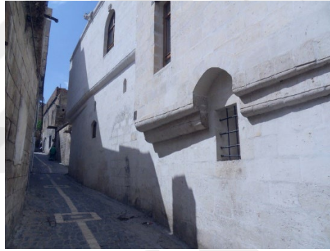
Figure 17: Nuran Elçi mansion south facade 2 (TEMA 2008: 21)
