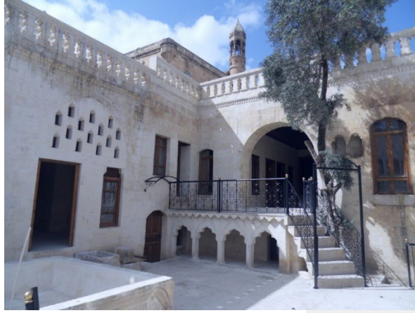
Figure 18: Nuran Elçi mansion courtyard north and west facades (TEMA 2008: 23)
