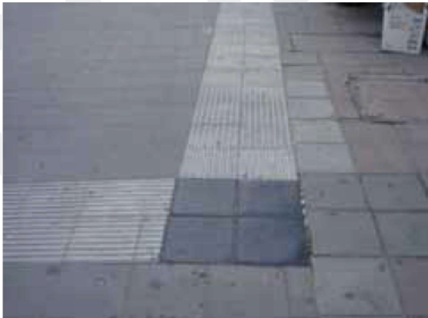
4.1.17. Rubber Warning Blocks Where Directional Blocks Intersect (Brussels, Belgium)
