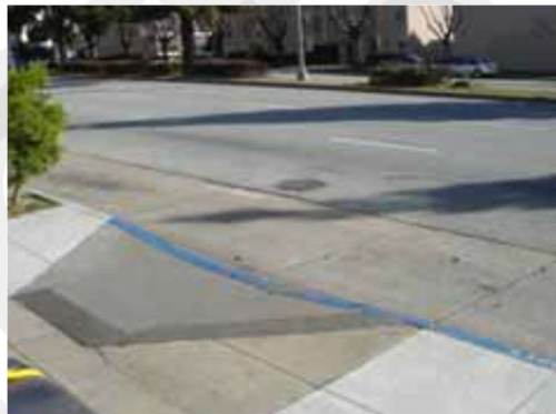
4.2.1. Shallow Grooves Cut into the Pavement before a Crosswalk (San Francisco, USA)
