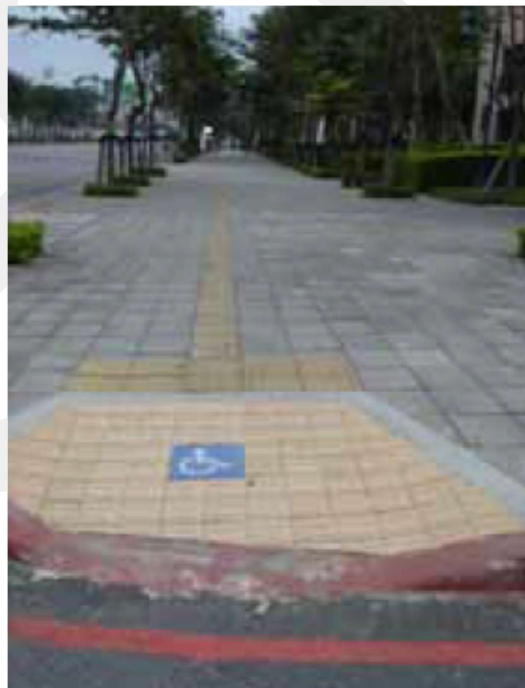
4.3.3. Blocks Installed Across the Sloped Area before a Crosswalk (Taipei, Taiwan)
