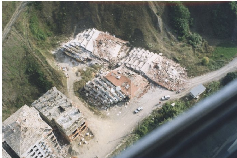
Figure 2.4. Buldings that are completely collapsed during an earthquake.
