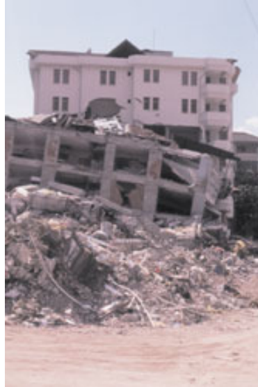
Figure 1.7. A completely destroyed building in front of a healthy building.
