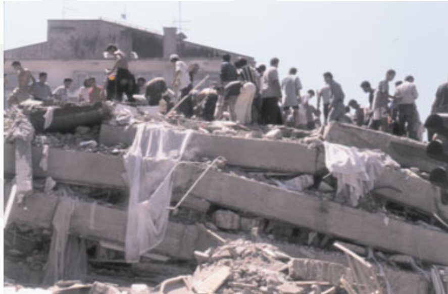
Figure 1.6. A completely destroyed building.
