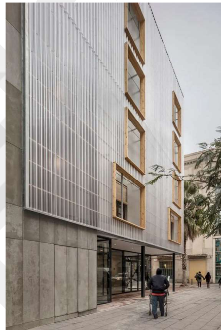
Figure 42. Façade Design with Polycarbonate Material. (Url 35)
