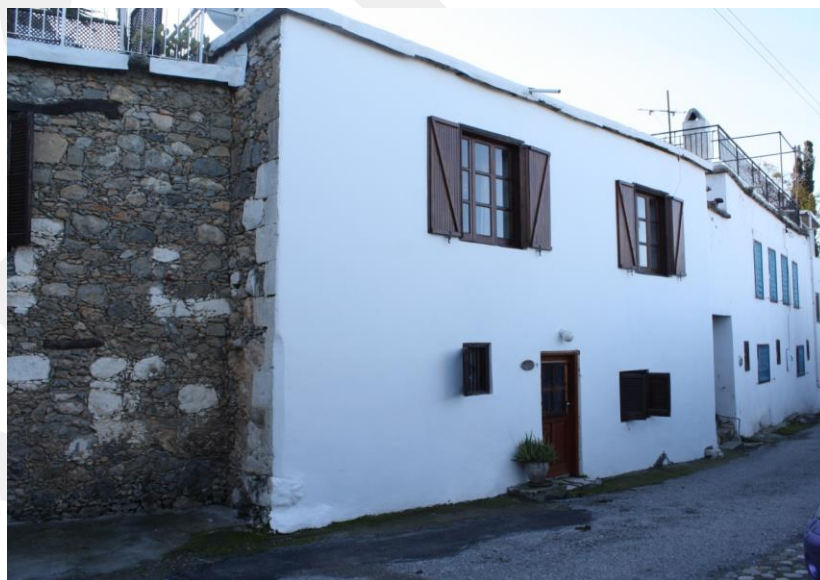
Figure 5. 11 Northside facade view of House One (Movahedi 2014).
