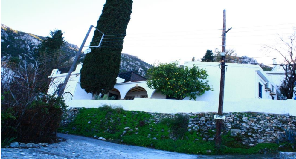
Figure 5. 15 Exterior Walls of House 2 (Movahedi, 2014)
