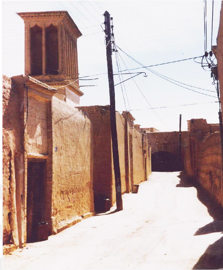
Figure 2. 8 Examples of structures that harness wind in order to decrease the use of nonrenewable energies and regular street pattern. Yazd, Iran (Movahedi, 2004)
