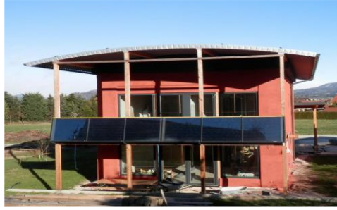
Figure 2.1: Passive House Ebner
