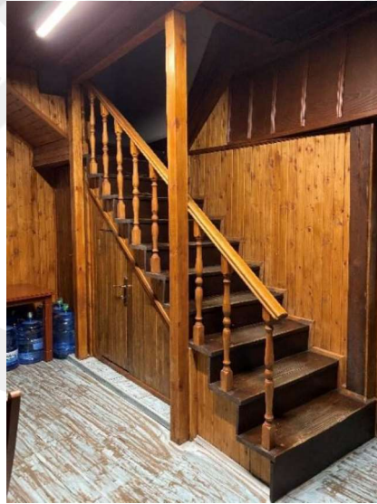
Figure 35. Hamamönü Region, Türk Kızılay Youth Center Building Street Rehabilitation Project Implementation Buildings Wood Staircase, Railing (Author's Archive, 2021)
