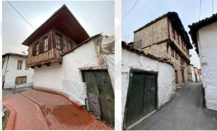
Figure 88. Traditional Buildings of Hamamönü, 2021 (Author's Archive)
