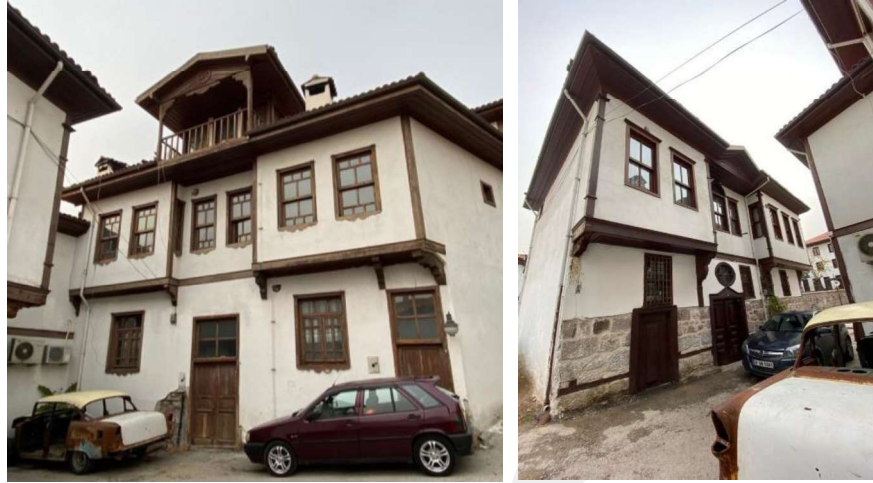
Figure 87. Traditional Buildings of Hamamönü, 2021 (Author's Archive)
