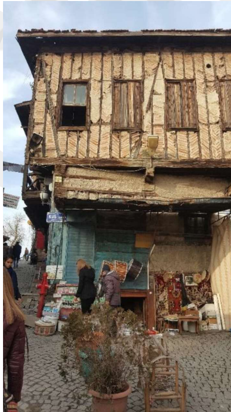
Figure 23. Ankara Castle Region, Ankara House Timber Framed- Brick Infill in Herring Bone Pattern (Author's Archive, 2020)
