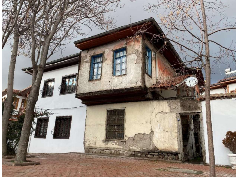
Figure 24. Hamamarkası Region, New and Old Buildings Side By Side Bay Window, Eaves, Stone Floor, Tile Cover, Window Iron Railing (Author's Archive, 2021)
