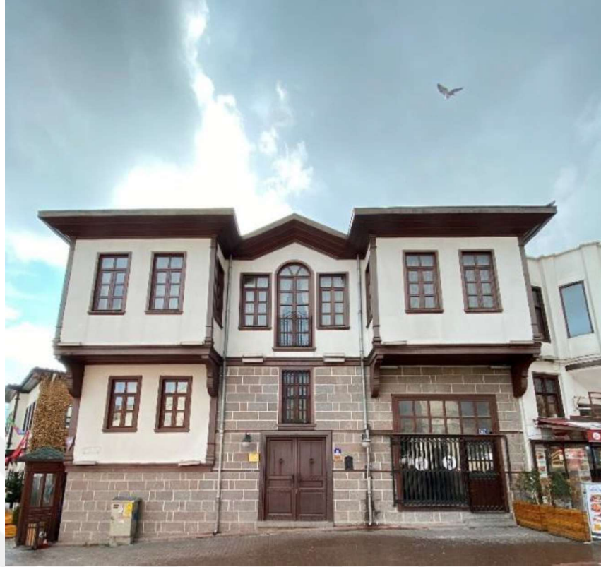
Figure 123. Kâmil Paşa Mansion, 2020
