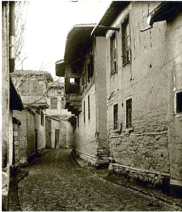
Figure 72. Hamamönü Houses (Undated)
