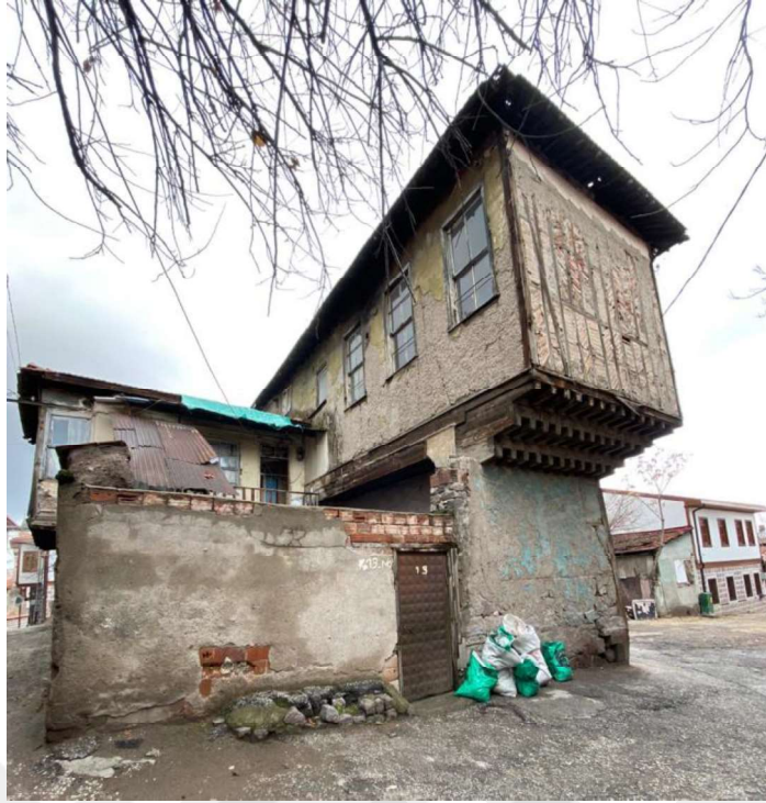
Figure 46. Ankara Hamamarkası Region, 3-Step Corbelling Bay Window (Buildings Photographed By Tuncer, Figure x.y) (Author's Archive, 2021)
