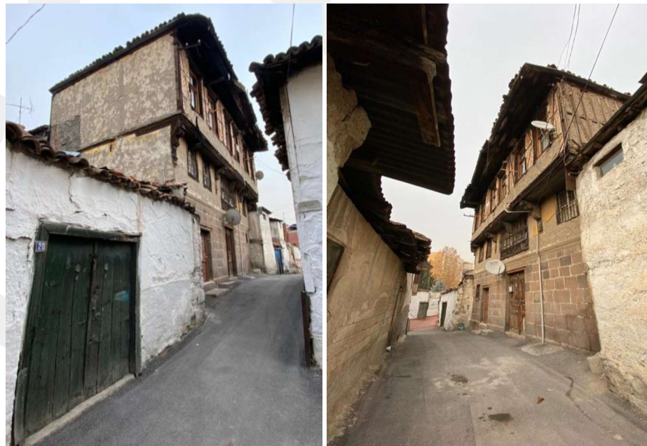
Figure 31. Hamamarkası Region, Old Ankara House) Ankara House and Mezzanine Floor and From End to End Cantilever (Author's Archive, 2021)
