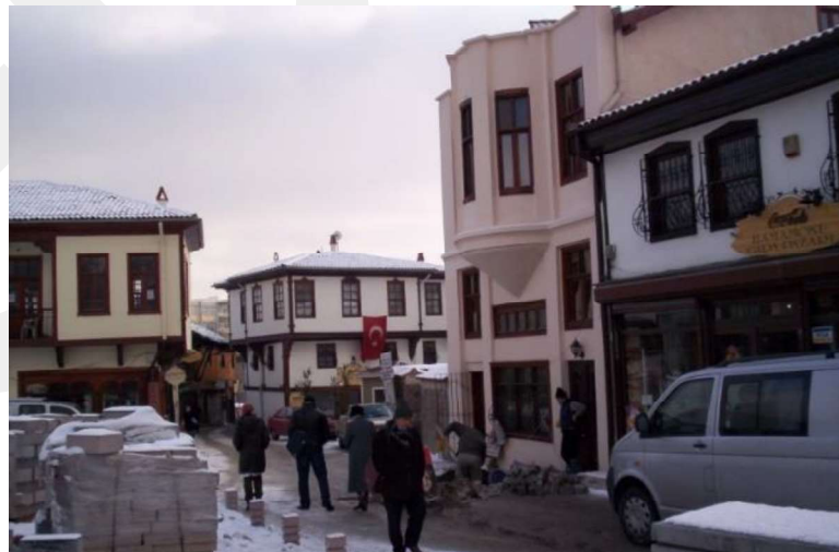
Figure 122. The Destroyed State of Kâmil Paşa Mansion, (Culture and Tourism Ministry, 2020)
