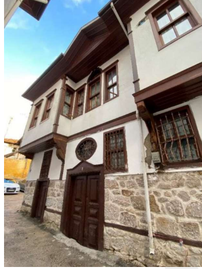
Figure 42. Hamamönü Region, Ankara House / Application of Westernization period of the 19th and 20th centuries Stone Ground, Mezzanine Floor, Simple Console Cumba ( Bay Window), Eaves, Iron Railing Window, Street Door, Door Top Elliptical Window, Floor Wiping, Gutter (Author's Archive, 2021)
