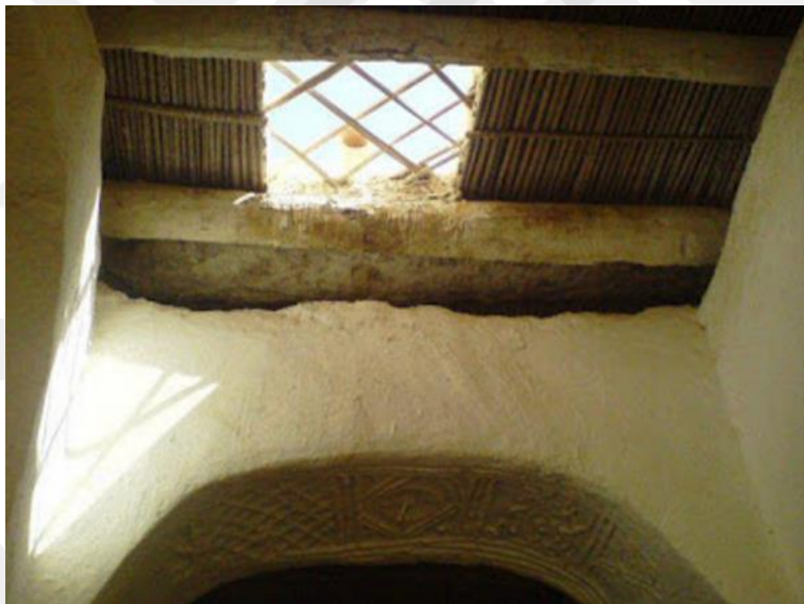
Figure 3.17: Natural lighting and ventilation openings at the roofs of the streets (Tinnaot) (Fteita, 2012)
