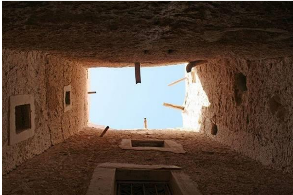
Figure 3.16: The big opening (Tinnaot) in between the houses' rears for ventilation and lighting at certain points at the streets(Researcher's collection)
