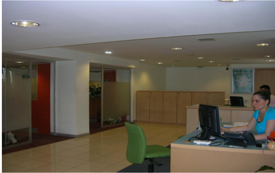
Figure 28: Garanti Bank recessed lighting fixtures in open office area (taken by the staff of Garanti Bank)
