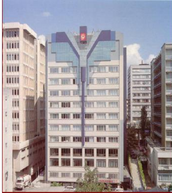
Figure 34: Pamukbank head office-facade of the building (Retrieved from www.google.com.tr/images )
