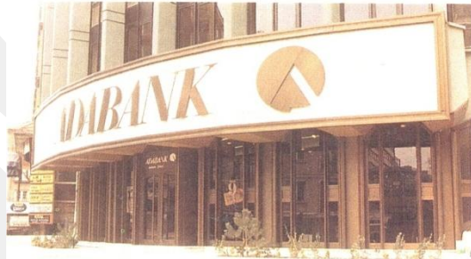
Figure 38: Adabank exterior facade
