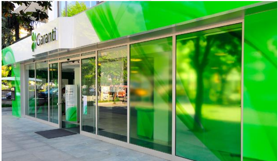
Figure 50: Garanti Bank new facade design
