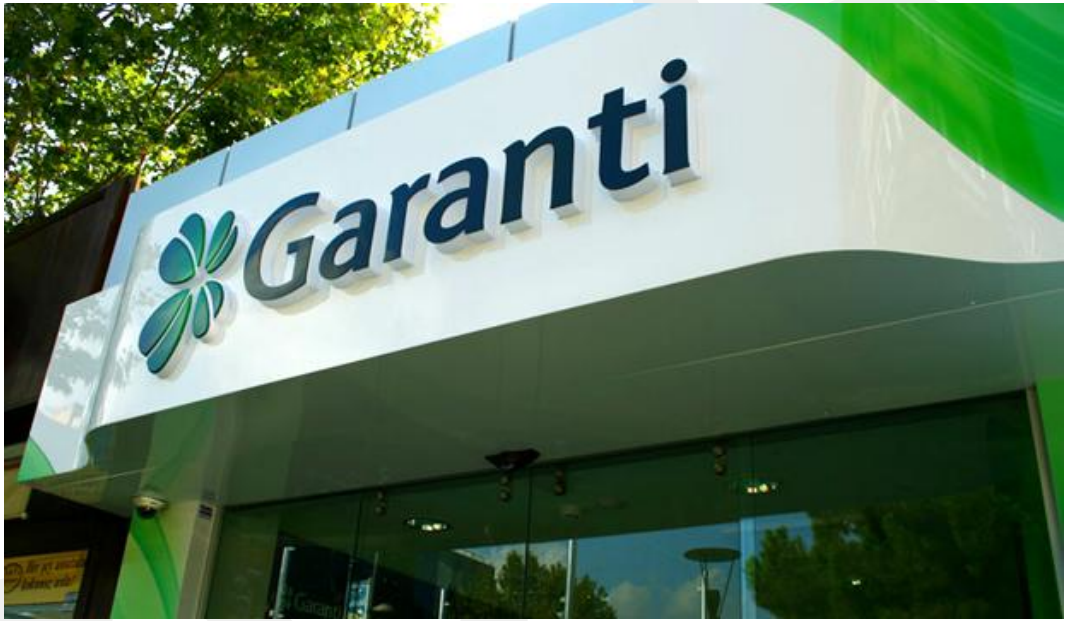
Figure 51: Garanti Bank new facade design
