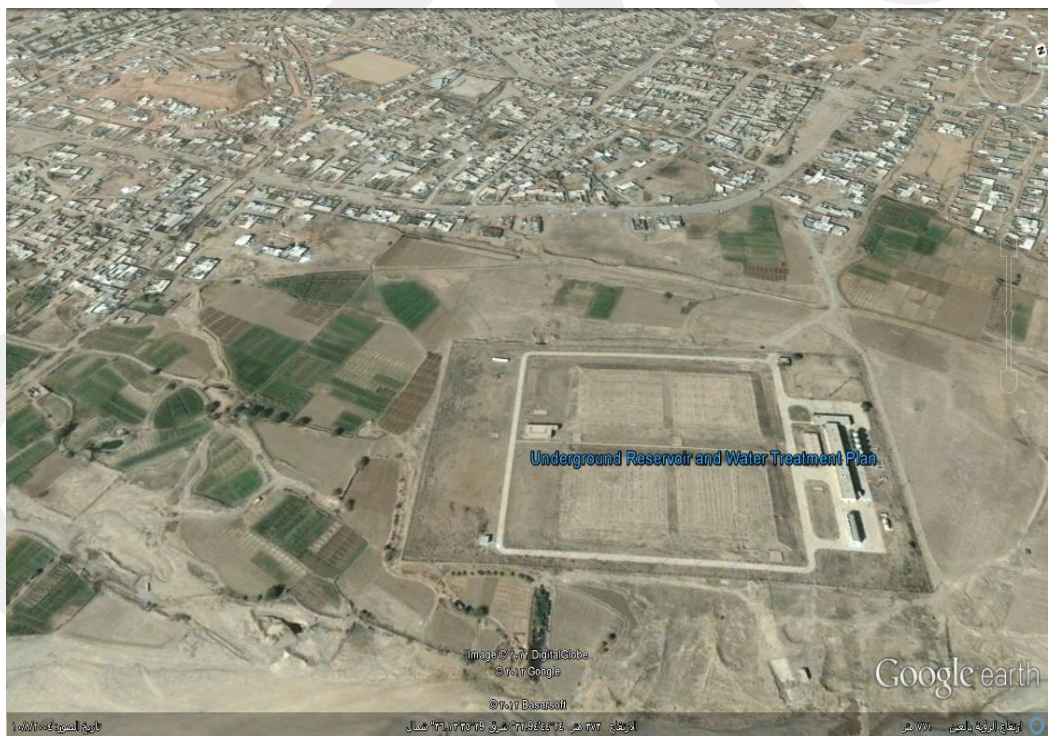
Figure 1.5 An underground Reservoir
