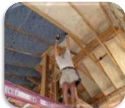
Fig 5.2. Cotton Batt Insulation (Hussein, 2012, p.6).
