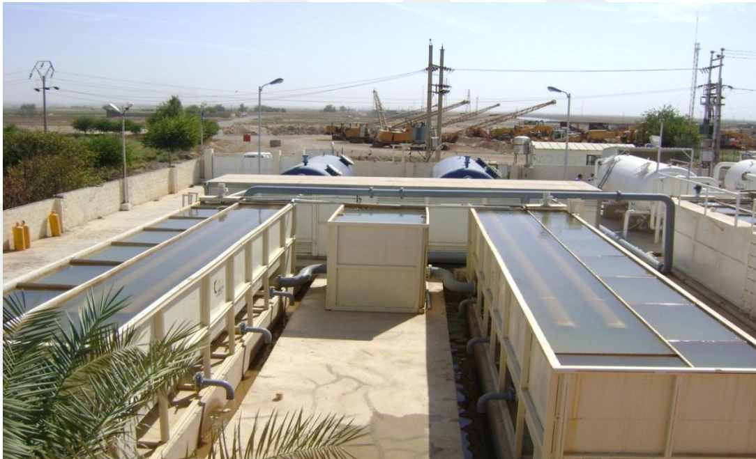
Figure 1.4 Compacts unit with capacity 200 \text{ m}^3/\text{h} used in Iraq-Kirkuk
