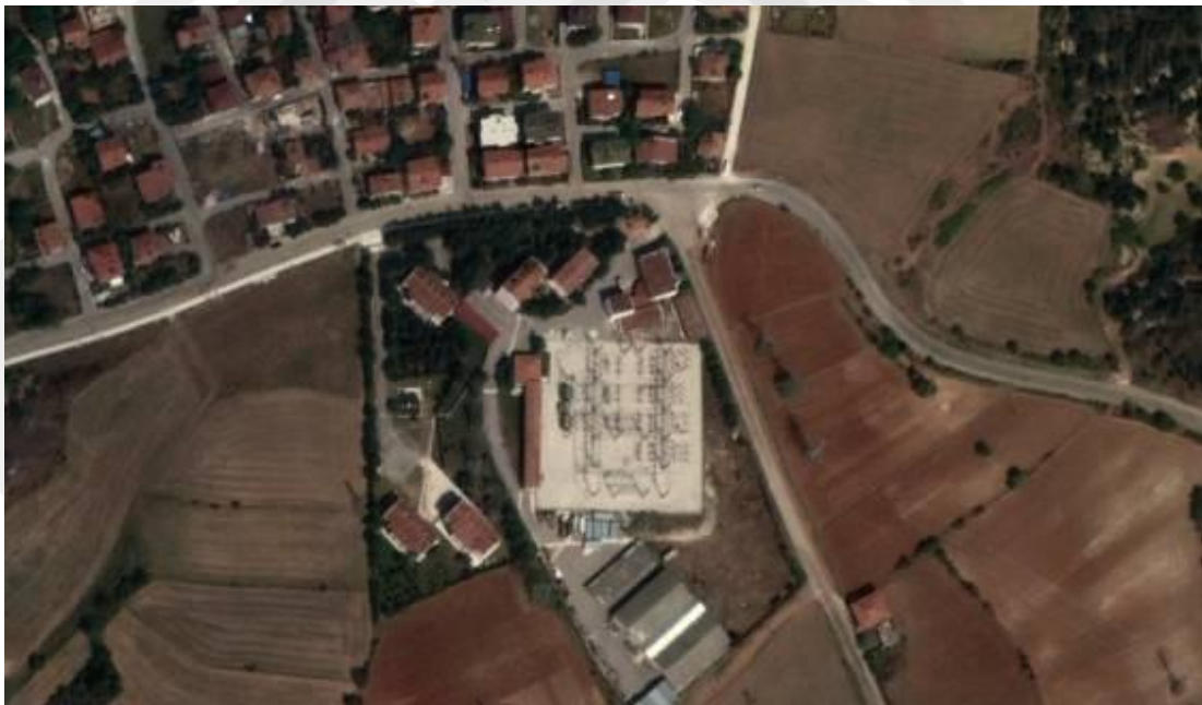
Figure 71 Top view of Kastamonu Substation
