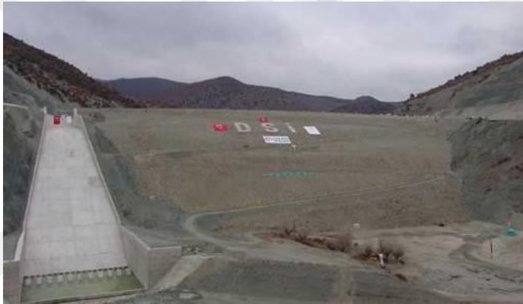
Figure 41 Karadere Dam, body and spillway
