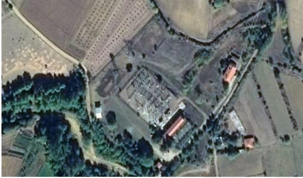
Figure 43 Top view of Taşköprü Substation
