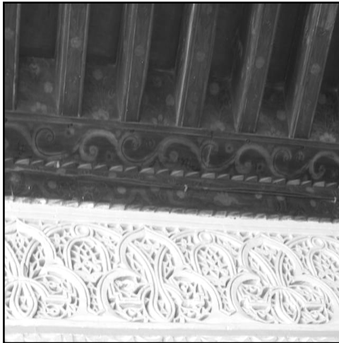
Figure 4.44 Ceiling of M. Gurgi Mosque 1834 (Samira.N.B.Said 2005)
