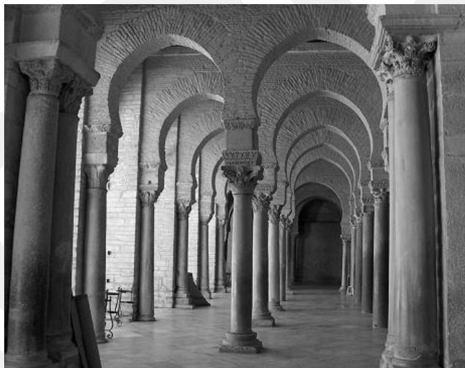
Figure 2.11 The Columns of the Prayer Hall are even Older, Roman and Byzantine Structures in Carthage and Hadrumetum (by Tore Kjeilen.2004)
