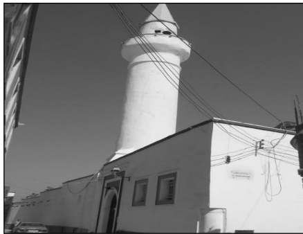
Figure 4.2 Exterior View of Dargut Pasha Minarat 1556A.D (Samira.N..B.Said 2005)
