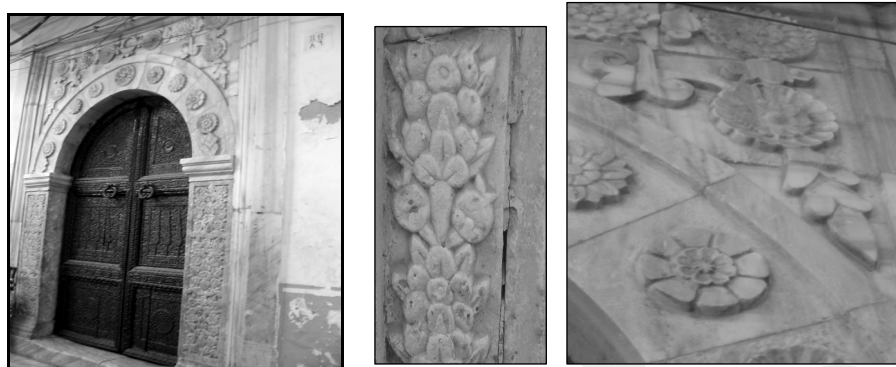
Figure 4.18 The Design Structures Such As Simple and Ornamental Pillars, Marble, Wooden of Southern Entrance of Mosque (Samira.N.B.Said 2005)
