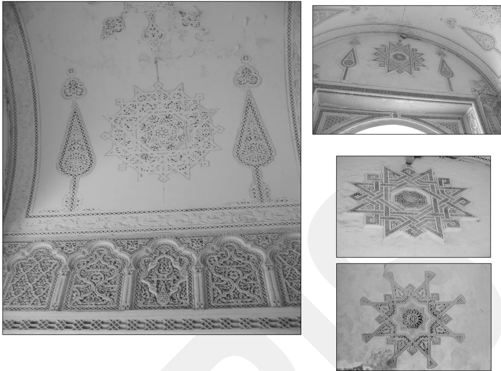
Figure 4.41 Technique of Decoration applied on Lime or Gypsum Surface in M . Gurgi Mosques 1833-1838 Is Typical of Qairawan, Tunisia, 837-875 (Samira.N.B.Said 2005)
