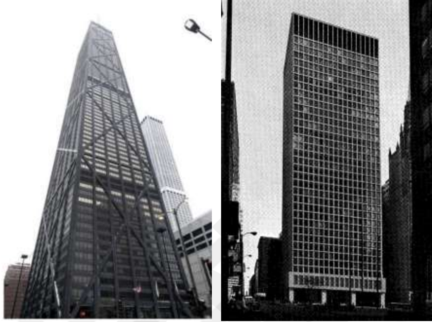
Şekil 2. 11: John Hancock Center (url-18), Brunswick Building (url-19)
