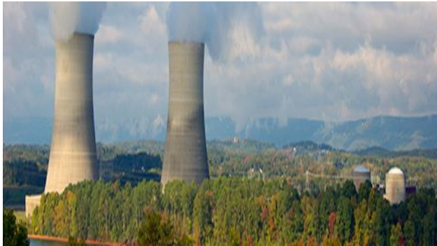
Figure 8: Nuclear Power Plant
